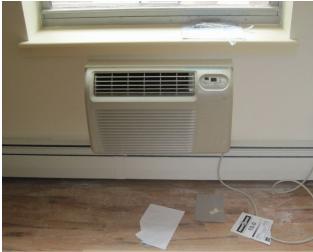
Fig. 4: Sleeve with AC installed
