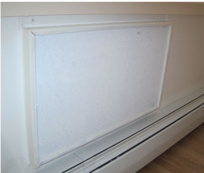
Fig. 11: Metal panel installed in Building 4
