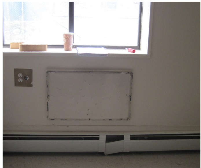
Fig. 12: Metal panel installed in Building 6
