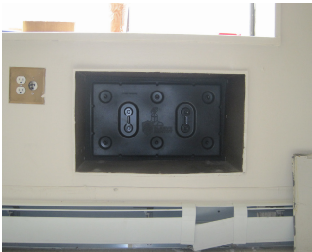
Fig. 17: Sleeve Sentry installed
